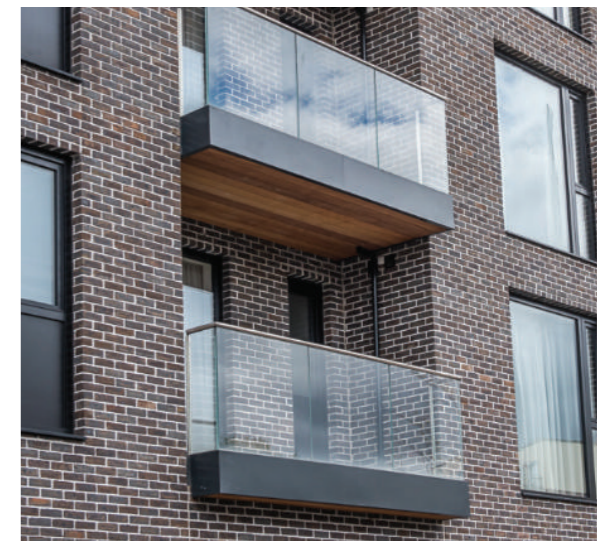
Glass balustrade to balconies
