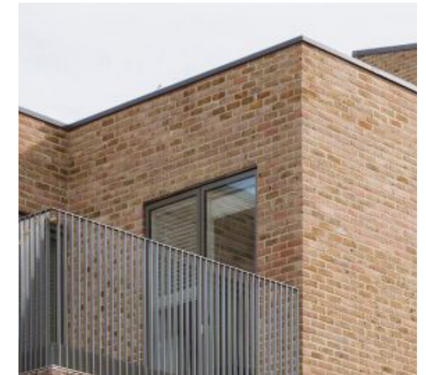
Dark metal windows and coping detail
