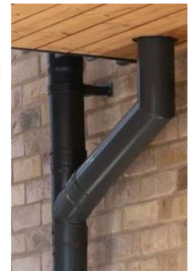
Drainage to the balcony
