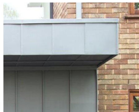
Metal entrance canopy
