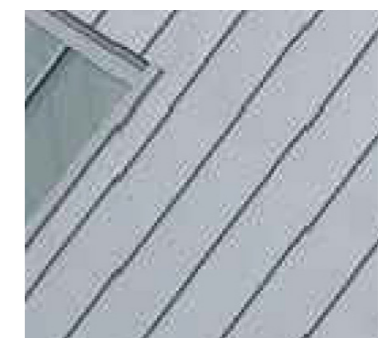
Metal cladding to stairs
