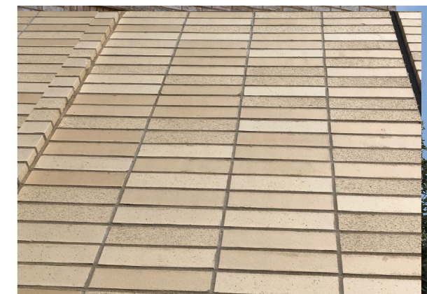
Stackbond brick detail to facade
