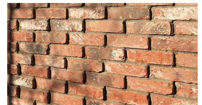
Stepped / protruding brick profile as seen in the walled garden
