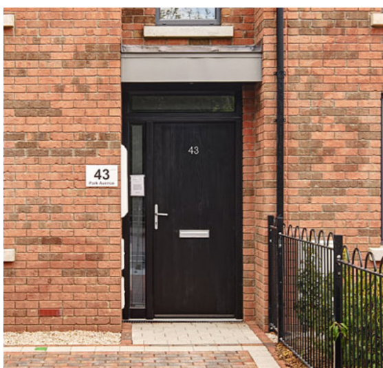
Painted timber entrance door
