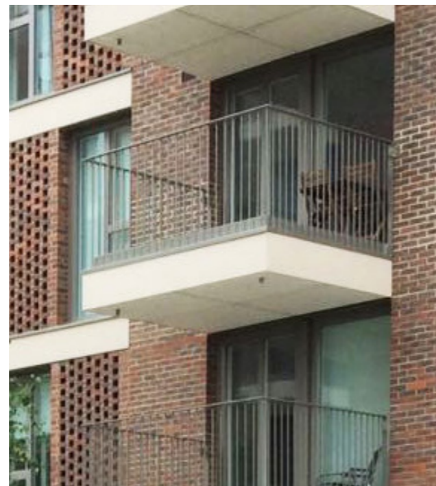
Example of glass cantilevered balconies
