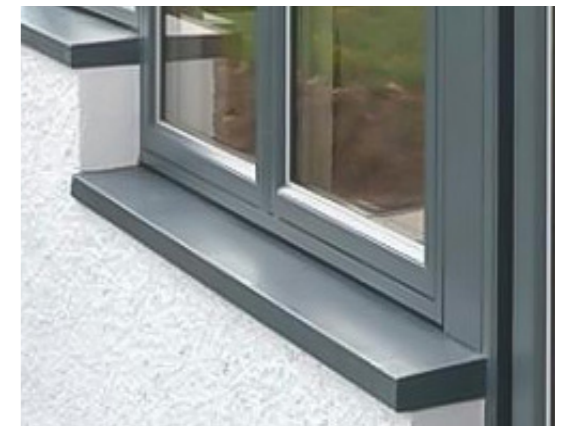
Pressed metal cill and window
