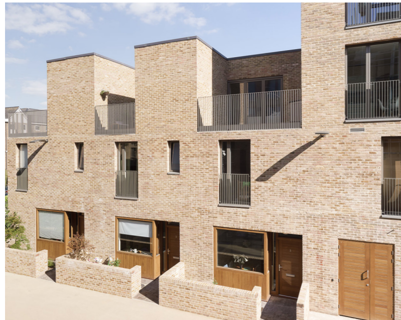
Recessed balconies with metal guarding Light ochre brick colour
