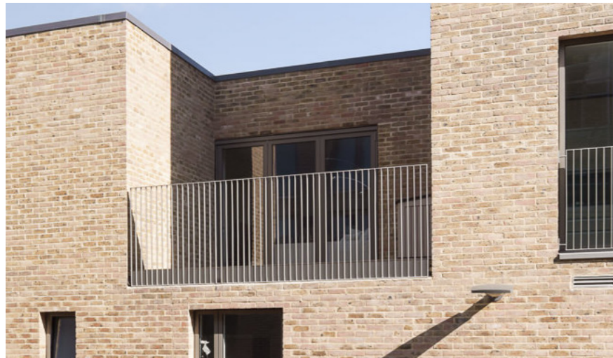
Powdercoated aluminium windows and metal guarding detail
