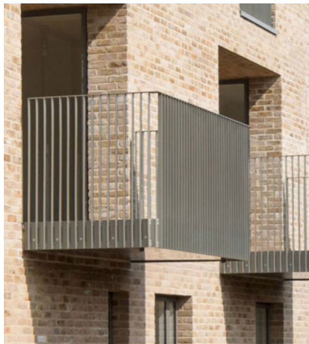
Example of metal guarded semi-recessed balconies
