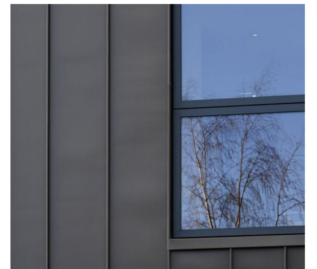
Dark metal cladding / window detail
