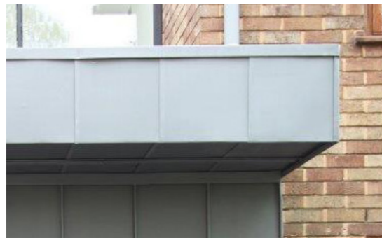
Standing seam metal entrance canopy
