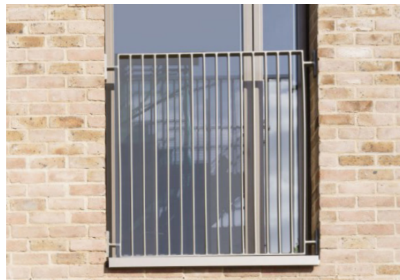
A dark metal Juliet balcony guarding used to the windows at first floor level.
