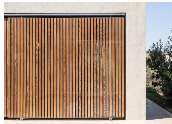
Timber slatted type doors to the communal areas on the north elevation
