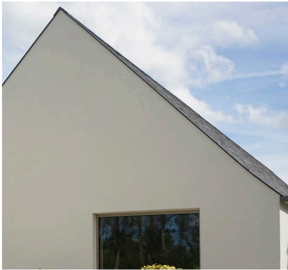
Flush eaves detail to roofs
