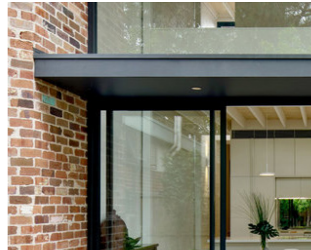
Metal entrance canopy
