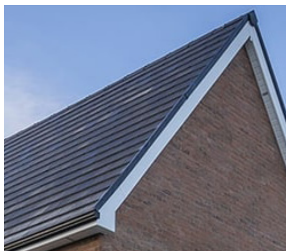
Dark concrete tile to roofs
