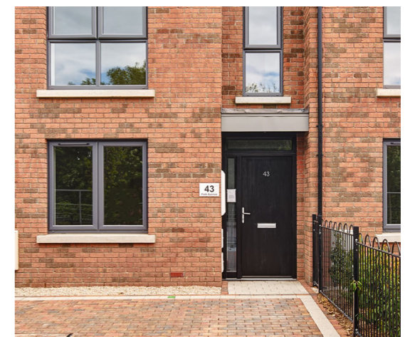
Painted entrance doors to own door units
