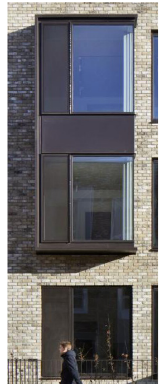
Metal bay window and brick detail.
